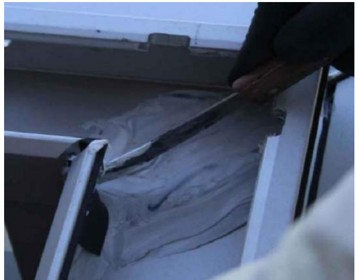
Apply weatherproofing sealant.
