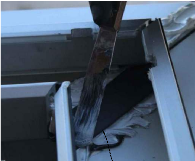
Install silicone splice membrane
