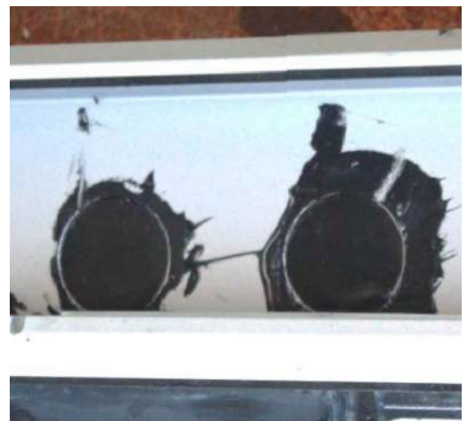
Tool sealant on access holes
