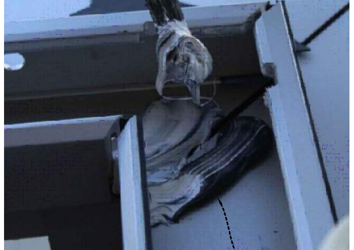
Apply weatherproofing sealant
